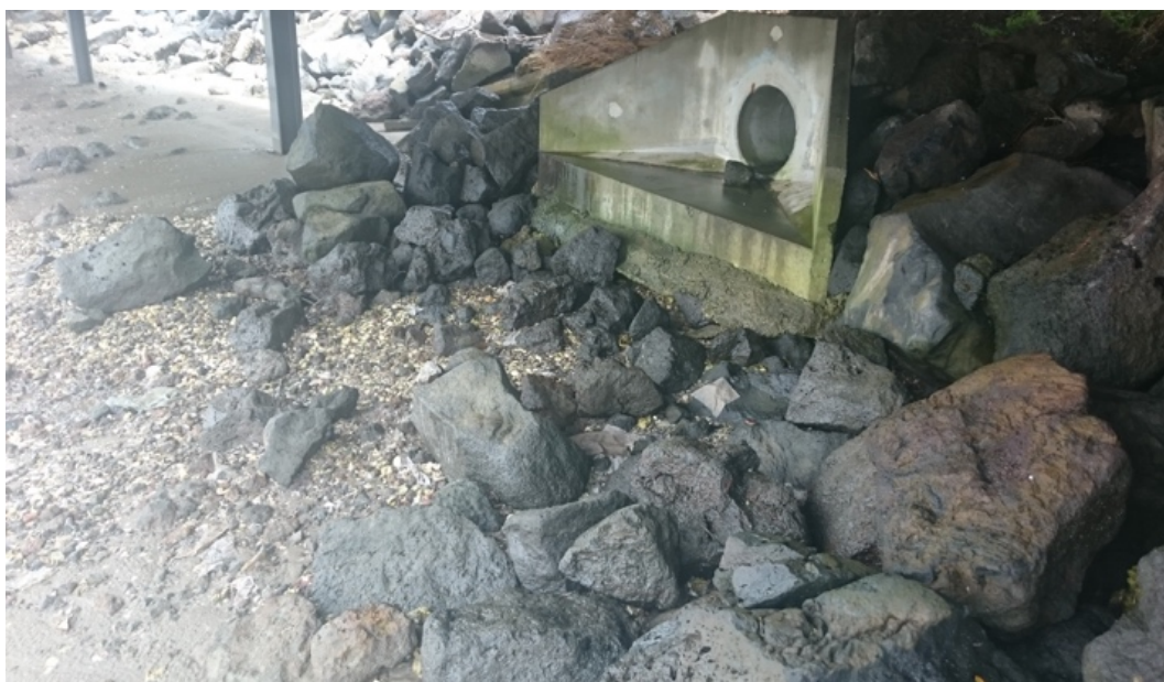
Figure 3. Combined Sewer Overflow to St Marys Bay showing debris resulting from its operation – odorous and visible at low tide (photograph taken 15/09/15).
