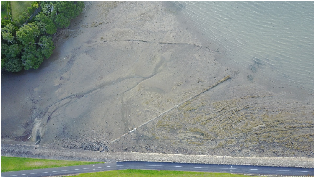
Figure 4. Existing pipeline at Masfield Beach (March 2017, Wilde Media Ltd).
